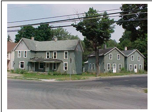
Before Photo by Larry Kilburn, Village of Arcade
